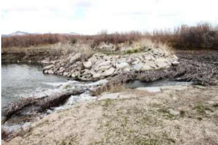
A diversion dam on the Humboldt River is containing a headcut
